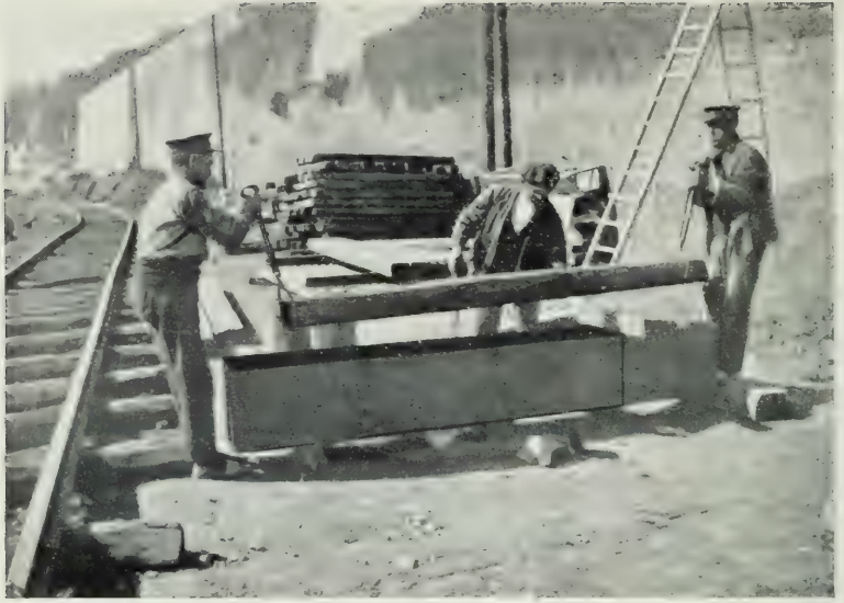
FIG. 115. DIPPING SLEEPERS IN "SOLIGNUM" TANK. [By courtesy of Messrs. Major & Co., Ltd.]
